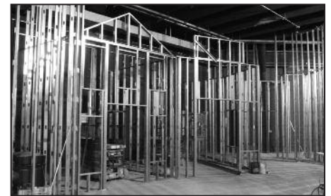
Walls are going up on the Energy City, photo above.
